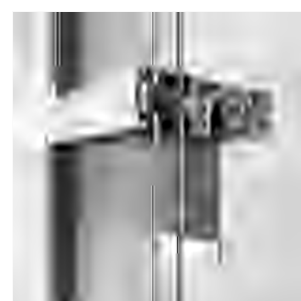
03 & 04 - Schueco FW550 Aluminium glazing facade system or equiv. (03) with integral blind system (04)
